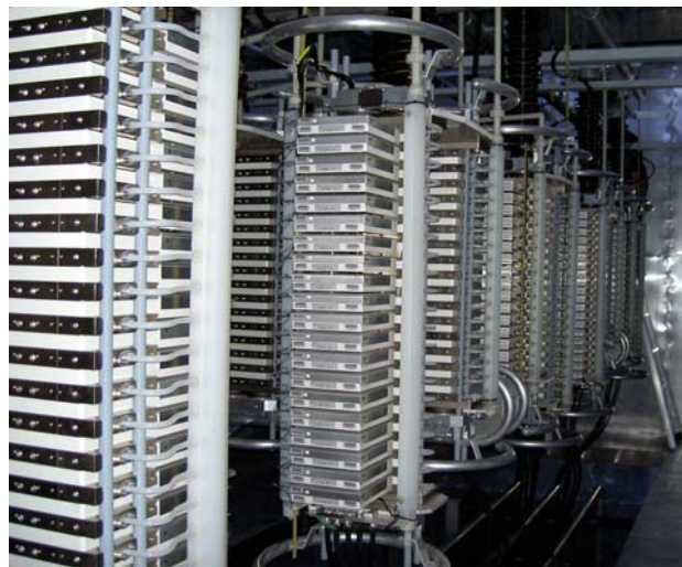
Fig. 3: Converter valve assembly.
