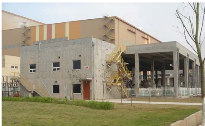
Fig. 5: Site view of the SVC Light.
