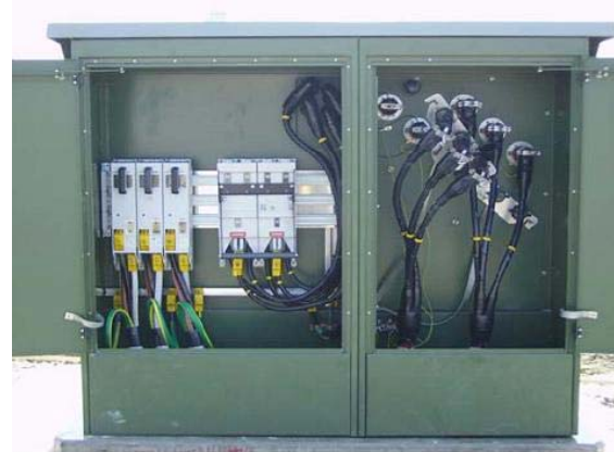
Figure 3. Transformer module (with or without internal P-coil)
