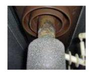
Figure 2- Example of degradation due to corona effect on field distributor on AIS switchgear.
