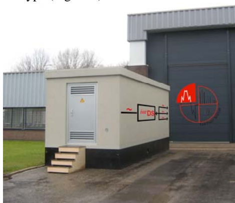
Figure 4 Smart substation in front of FPGLab
