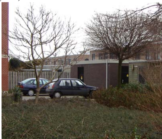
Figure 6 Substation on field trial location
