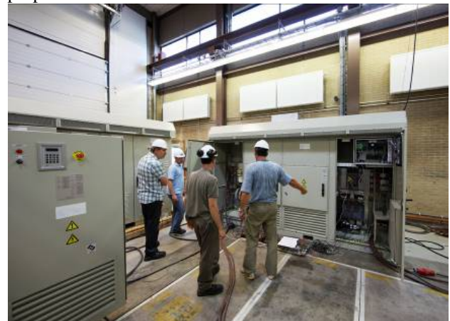
Figure 3 A range of utility-interactive PV-inverters undergoing testing in the FPGLab
