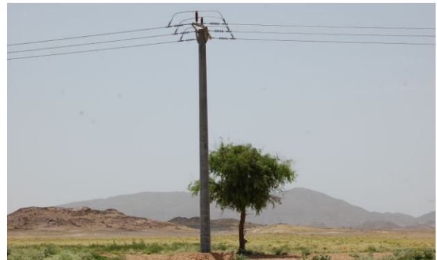
Fig. 1: MV angle section pole in the desert of Oman.
