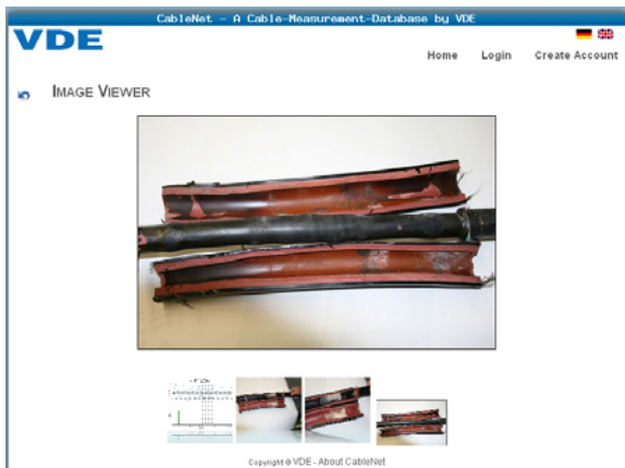
Figure 3. Image Viewer – pattern and pictures of visual inspection
