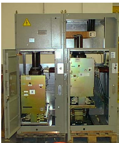
Figure 2: Enel compact type MV switchboard
