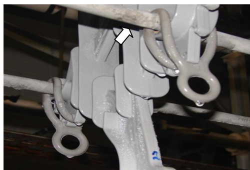
Figure 3 – Tracking and erosion in a covered cable.
