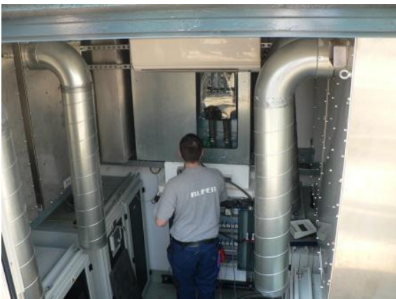
Figure 4. Interior of the SSU as seen through the main access door.
