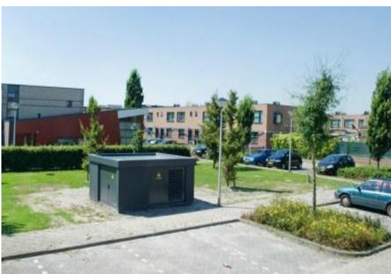
Figure 5. The SSU after installation on site in Etten-Leur.
