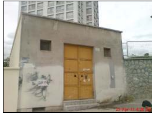
Figure.9: Typical substation Building
