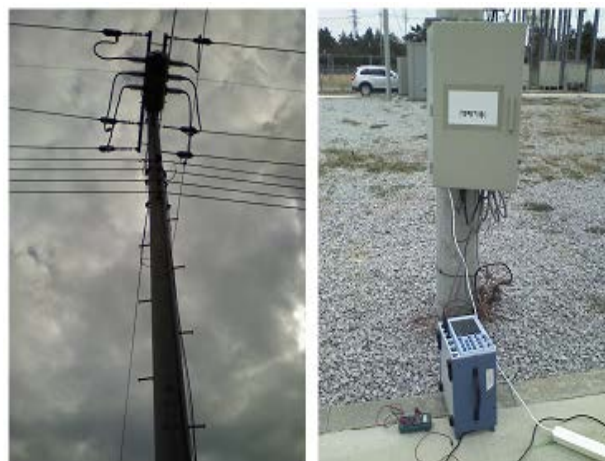
Fig. 2. Measurement of switchgear voltage error
