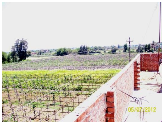
Figure 4. The overhead power line location in Case study II
