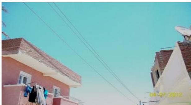
Figure 2. The overhead power line location in case study I
