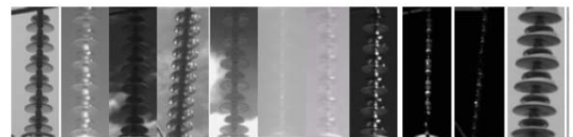
Fig.3 Zoomed in scenarios of outdoor insulator images. Left to right: sunny; sunny with reflection; 3 non-uniform cloudy backgrounds; 2 blurred images due to foggy; 3 images in dark nights; insulator covered with snow.
