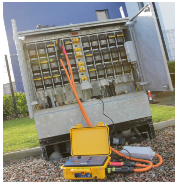
Figure 1- REZAP Fault Master Installer
