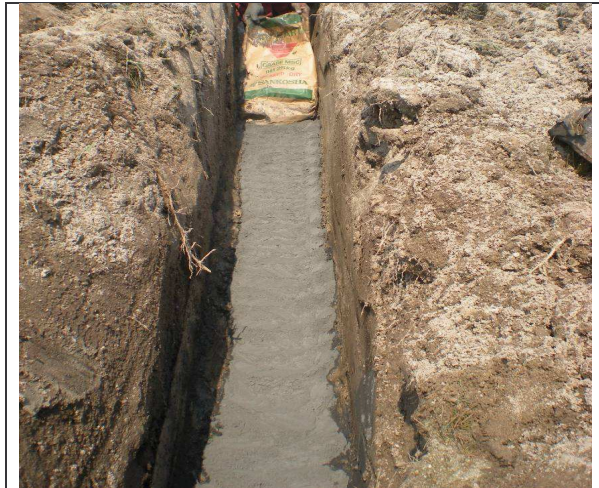
Photo 3: Applying Earth Enhancing Compound
