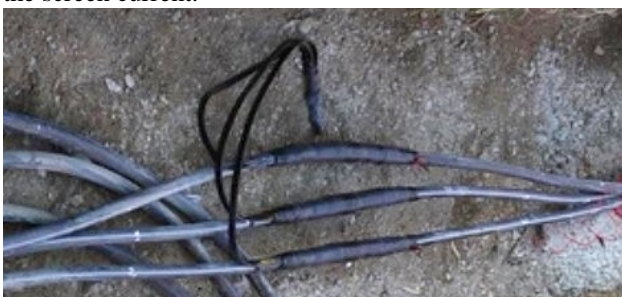
Fig. 1: Interconnection of the screens
