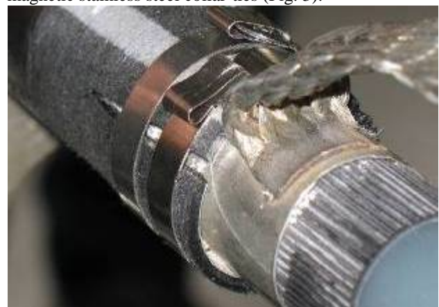
Fig. 3: Screen plate installed on the cable
