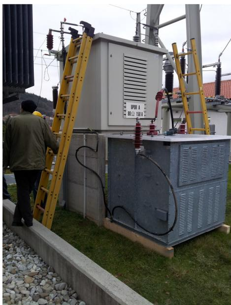
Figure 2: Field test site with existing NGR and additional NGR of 80  $\Omega$  resistance
