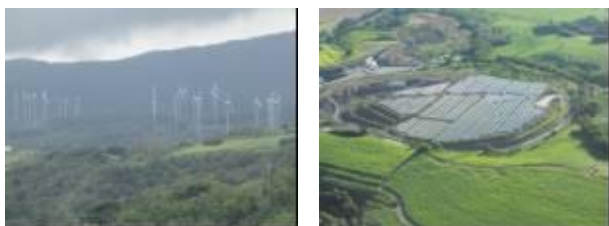
Fig. 4a - 10 MW wind farm Fig.4b - 2 MW PV farm
