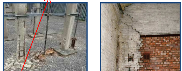
Image 1 – Major supports and buildings scored as HI5 in condition based assessment
