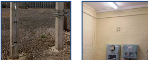
Image 2 – Major supports and buildings scored as HI2 after civil refurbishment works
