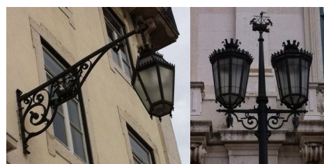
Picture 5 – Refurbished historical building lanterns.
