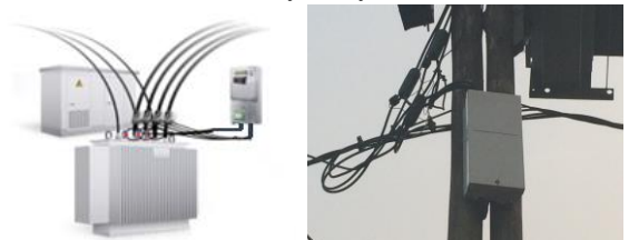
Fig.2 DTM meter in indoor and outdoor MV/LV station
