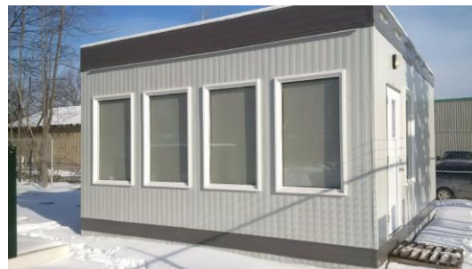
(a) MG control room
