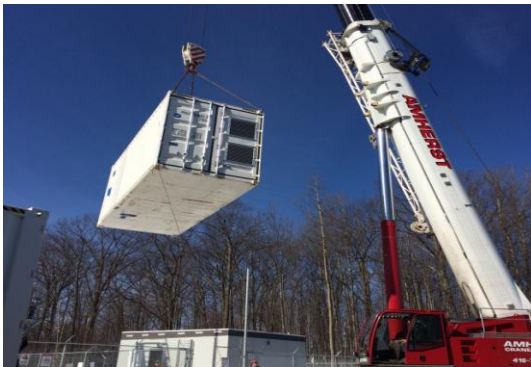
(c) Installation of ESS/PCS Fig. 6. Photos of site construction
