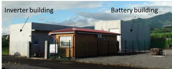
Figure 3. Storage system in the PEGASE project
