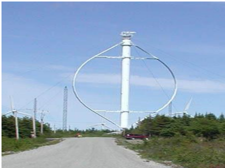
Figure6. A Vertical Axis wind turbine
