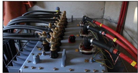
Figure 7: Transformer connections (left: LV, right: MV)
