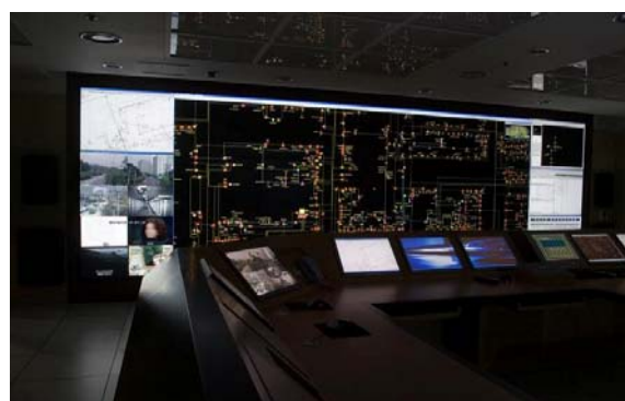
Figure 2 New Distribution Control Center
