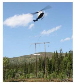
**Fig. 11:** from paper 1393 – Helicopter used for transport and placing of pre-assembled poles
