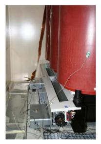
**Fig. 29:** from paper 0625 – Radial ventilation system at the bottom of a dry-type transformer
