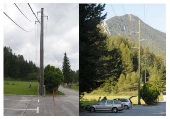
Fig. 15: from paper 0294 – Line before and after uprating from 35 kV to 110 kV
