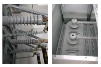
**Fig. 14:** from paper 0694 – RTV silicone application on insulating surfaces
