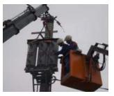
**Fig. 35:** from paper 0521 – Installation of a pole-mounted dry-type distribution transformer
