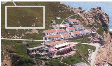
Figure 3: Approved area for PV installation in 2010
